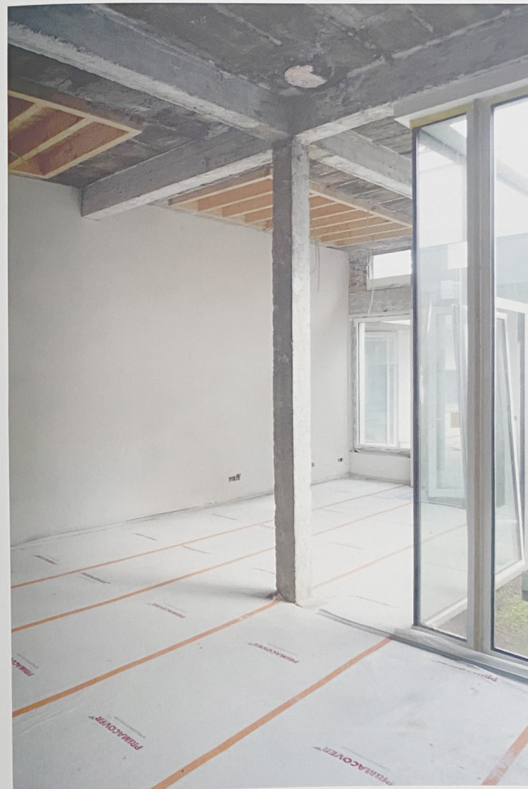
View of the interior and lime plastering
