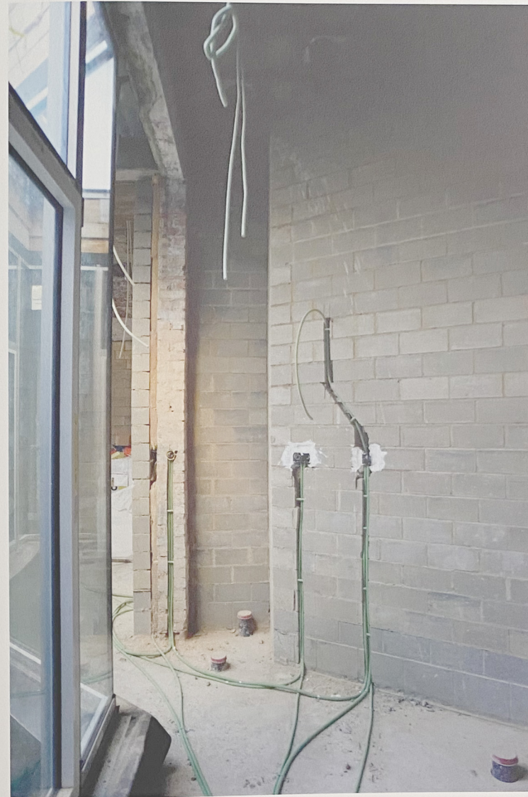
The earth block masonry during construction
